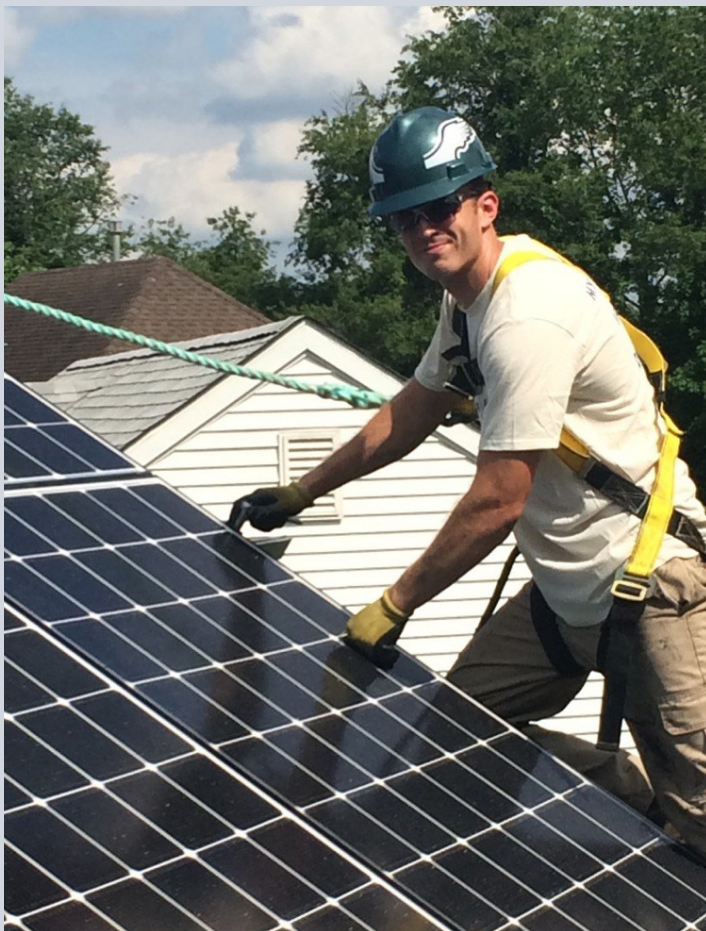
Michael Skala of Yardley, Pa.-based Exact Solar installs a solar array on a residential rooftop. (Photo courtesy of Exact Solar)
